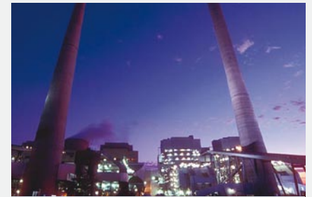
CS Energy's Callide Plant in Queensland
