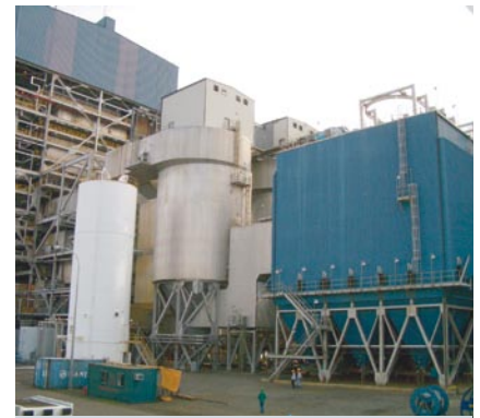
Power plant at Quezon
