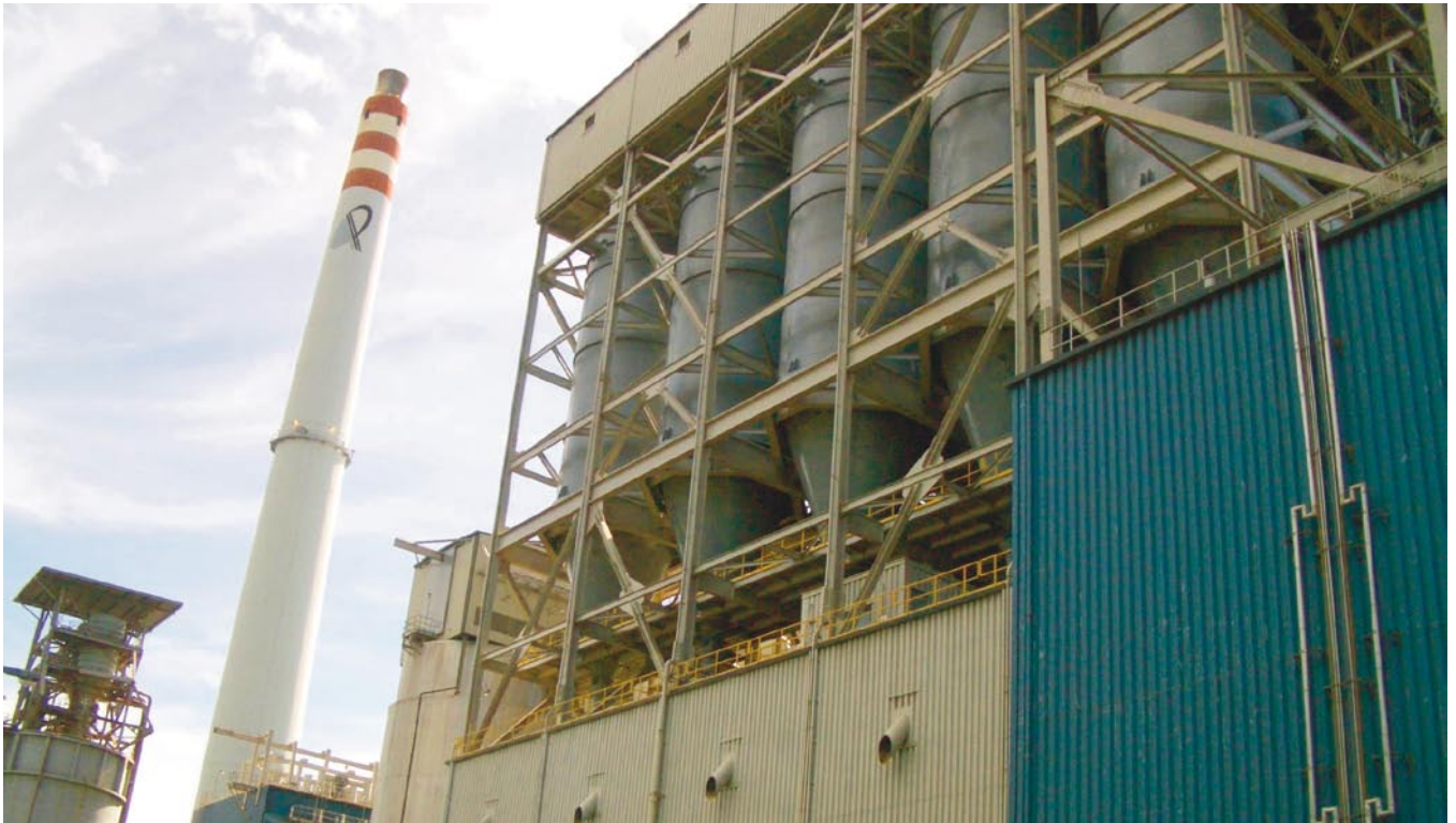
Quezon Power Limited's 470MW Quezon Power Station
