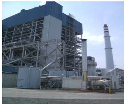
QPL's 470MW Quezon Power Station
